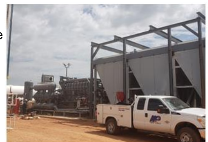
After Conversion - Installed in Field
